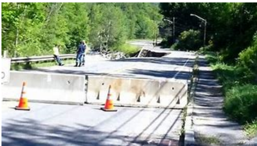
Figure 4: River Rd/Route 8 Damage from T.S. Irene
